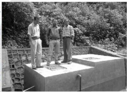
recommended that at least once in a month, the filter chamber is washed and cleaned. Chamber does not get damaged, this also has to be checked in small intervals of time.
